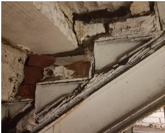
Existing Stair Support
