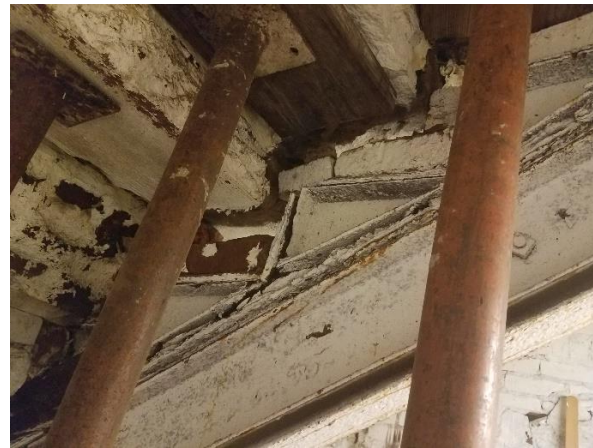
Existing Stair Support
