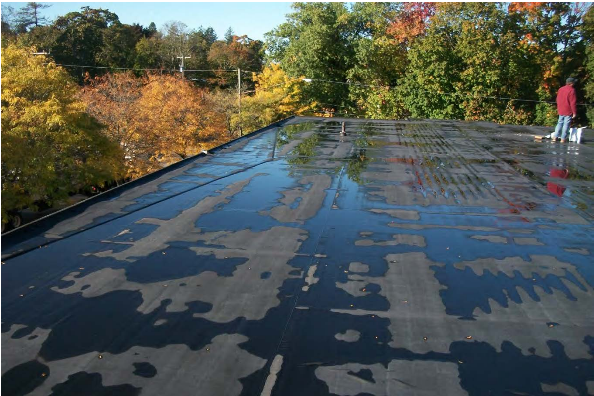
Building addition roof
