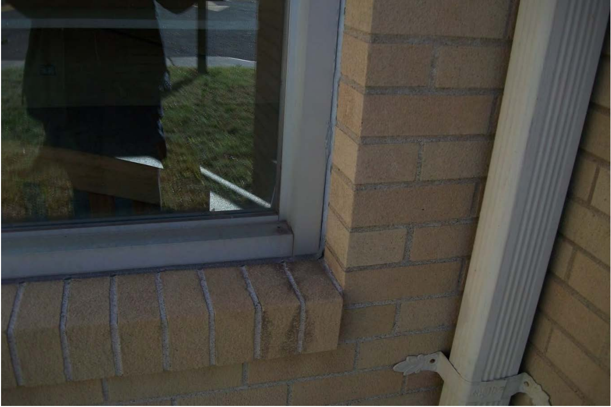
Representative exterior window caulking and glazing compounds
