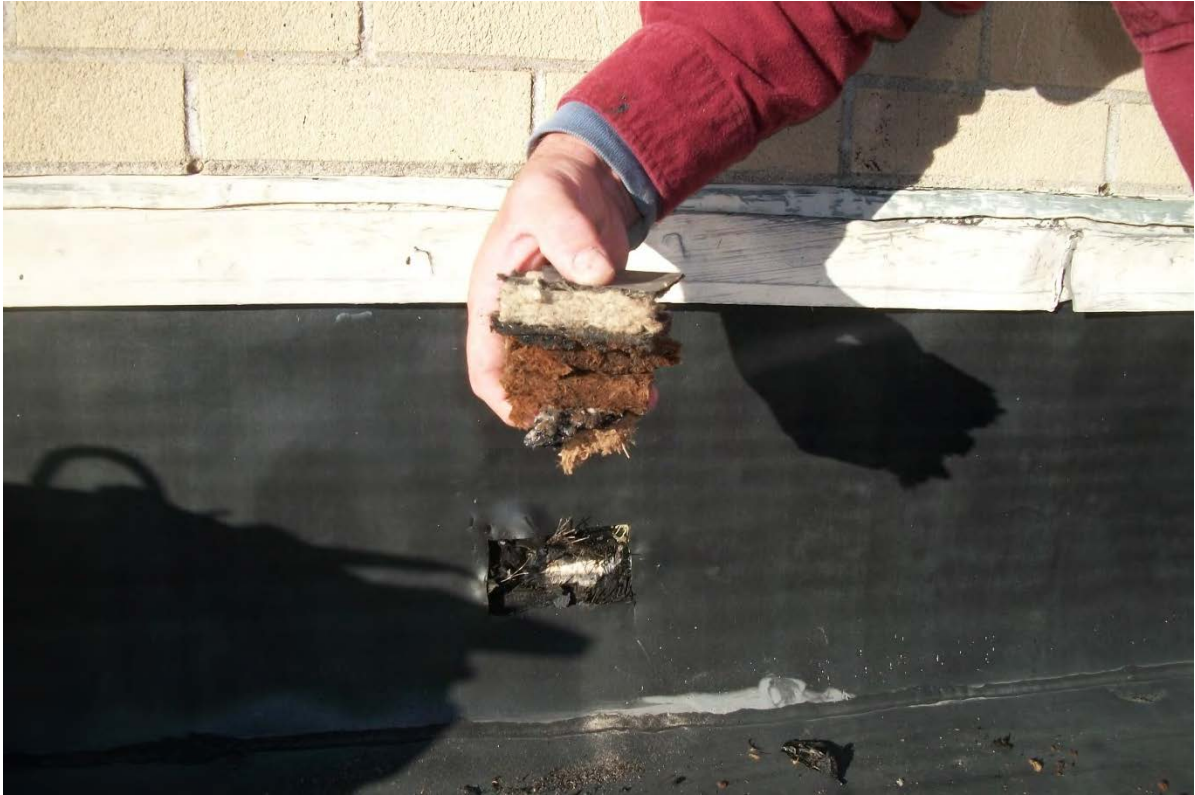
Connector roof composition
