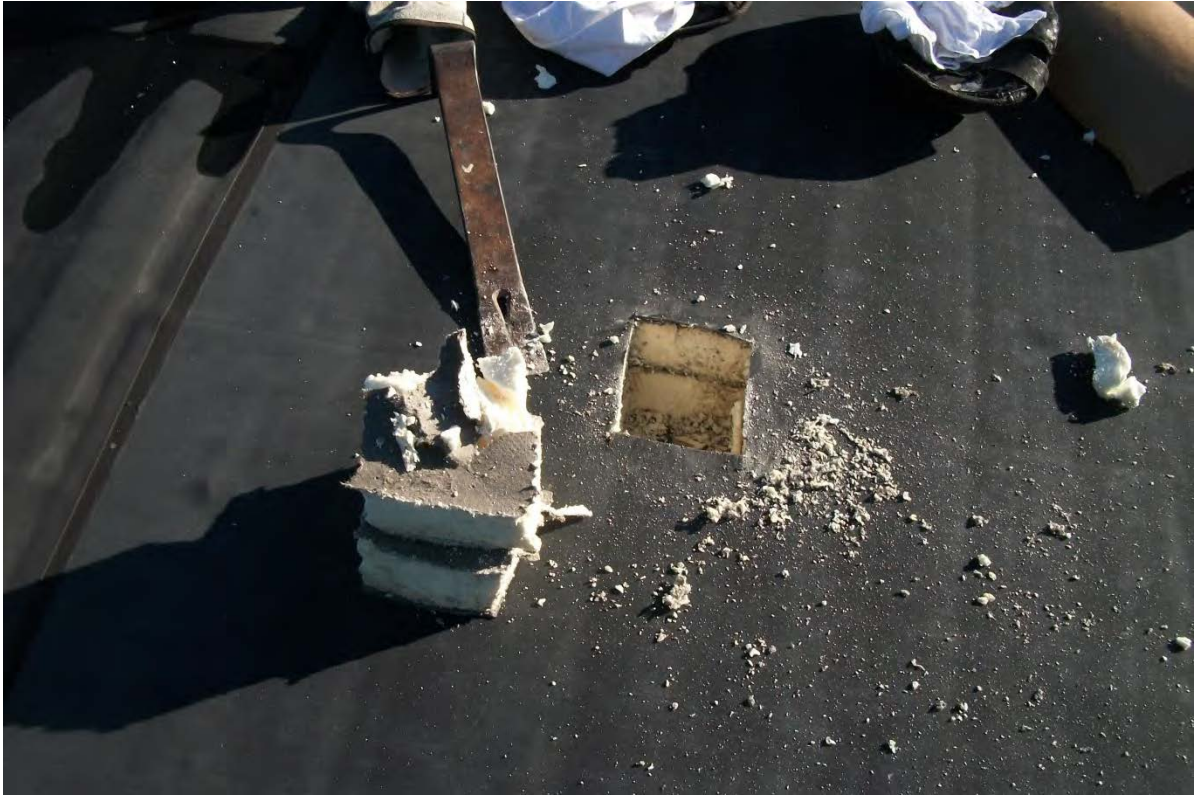
Building addition roof composition
