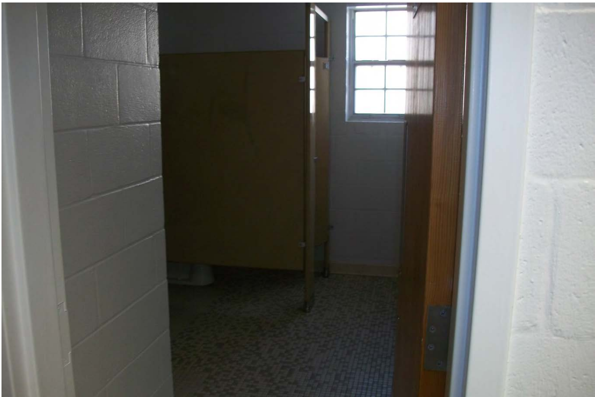
Building addition representative bathroom
