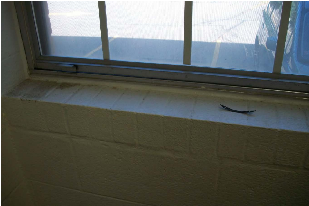
Representative interior window caulking and glazing compounds
